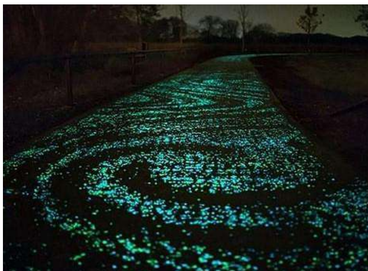
Fig. 9. Bicycle path made of light-generating cement [17]
